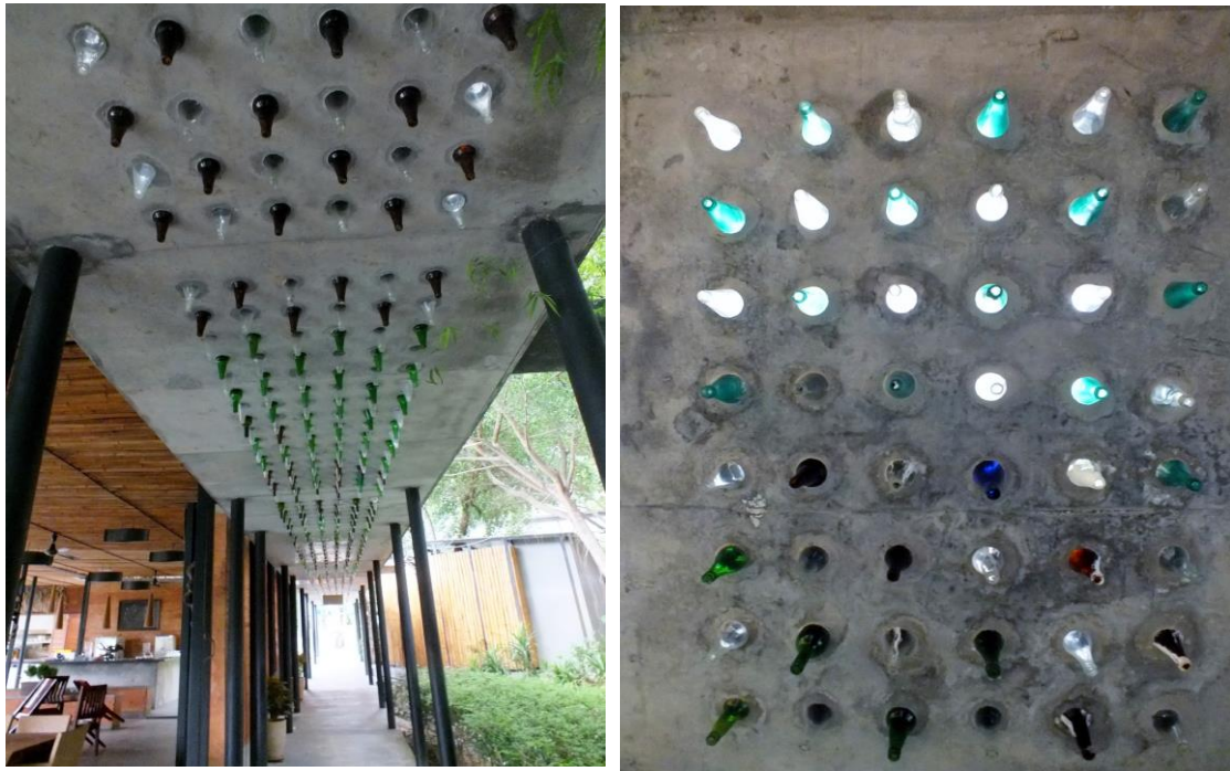
Photo 07 Bistro Walkway, Recycled Glass Bottle as Skylight
